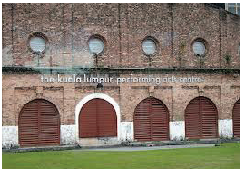
Figure 5 Exterior façade of KLPAC (original structure)
