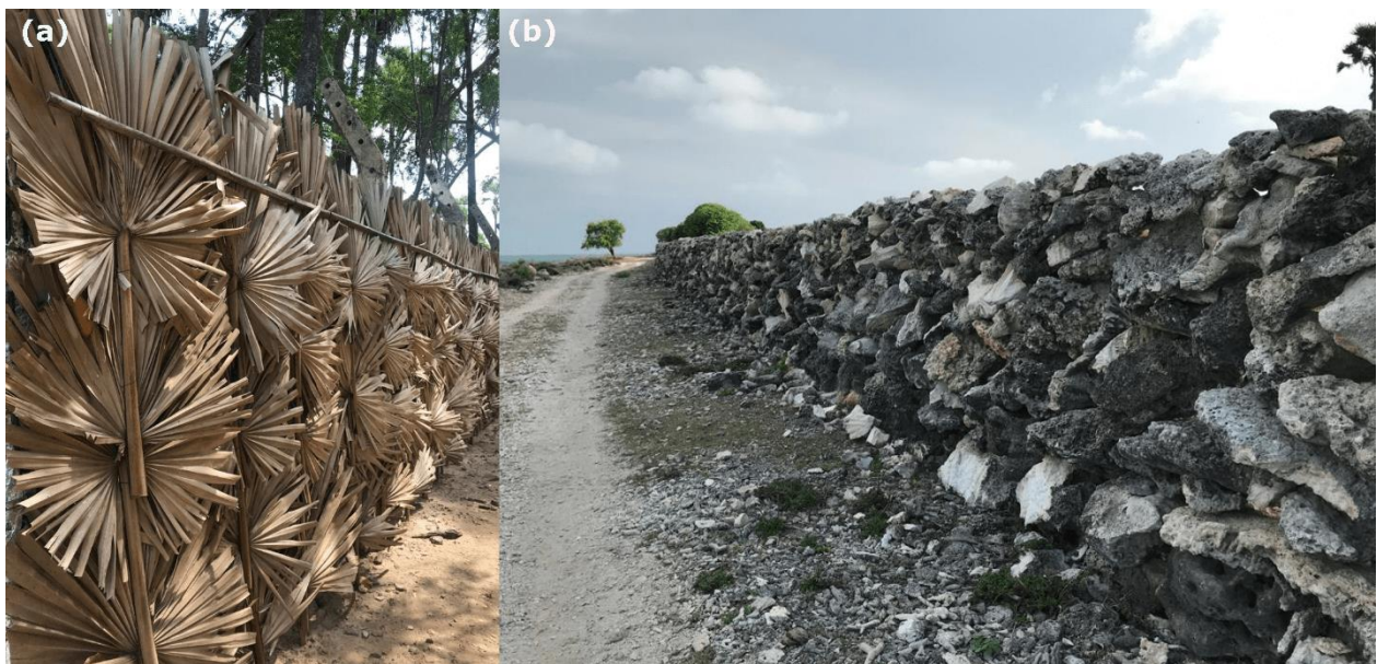
Figure 12. Traditional Walls Unique to the Jaffna Peninsula (a: Palmyra Leaf Wall in Jaffna; b: Coral Stone Wall in Delft Island)
